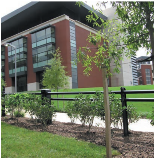
The cable is encased in the bracing rail. Other cables can also be run through the rail.
