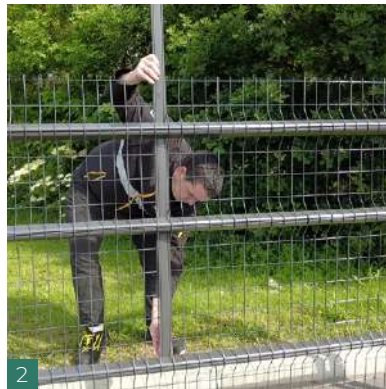
2 Secure the reinforcement elements by fitting a rigid slat in the middle of the panel. Repeat the operation on the other side of the panel.
