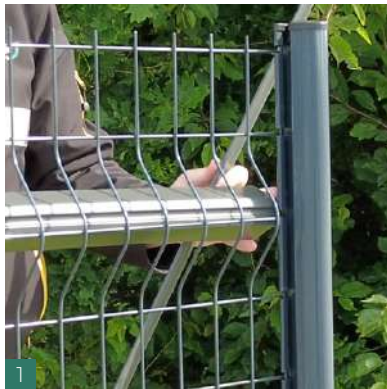
1 Position the reinforcement elements in the panel folds.
